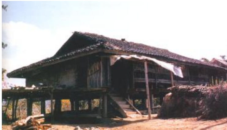
The resident features— The bamboo house with four eaves for draining rainwater
